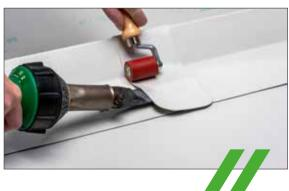
directly to the sheet metal by welding. Where the sheets are butted together, they are connected with strips of KÖSTER TPO U at least 10 cm wide. This is completely welded
