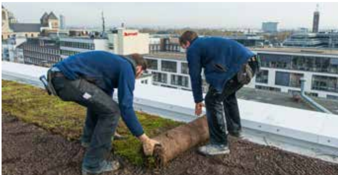
Installation of the green roof construction
