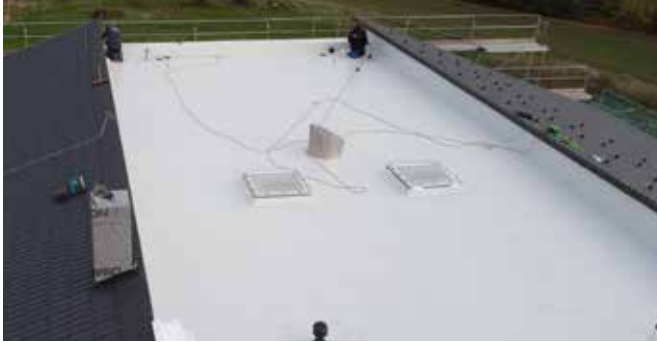
Installation of KÖSTER TPO waterproofing membranes
