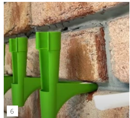
6 Insert the end of the capillary rod into the suction angles' supply tank and then push the capillary rod and the suction angle together into the drill hole so that the suction angle is securely stuck in the hole. The suction angle is reusable. The KÖSTER Capillary rods are not prewetted.
