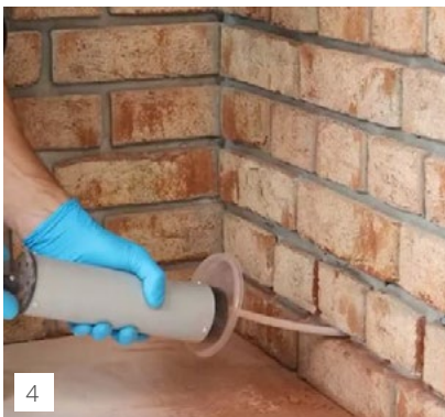
4 Clean the holes with KÖSTER Drill Hole Cleaner or flush with water.
