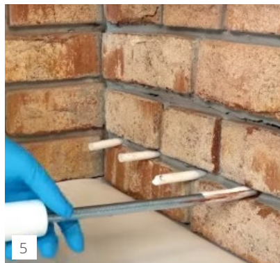
5 The length of the capillary rods must be at least 7 cm longer than the depth of the drill hole. Measure and cut the capillary rods accordingly.
