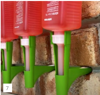
7 Place the KÖSTER Crisin 76 cartridge in the suction angle's clamping device, so that the supply tank fills up with KÖSTER Crisin 76.
