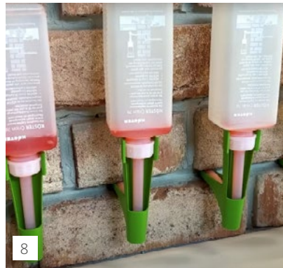
8 The cartridges remain in the wall for up to 7 days.
