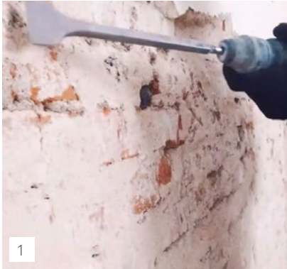
1 First the old damaged plaster is removed from the masonry
