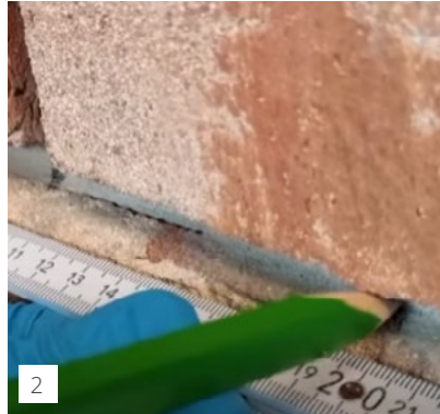
2 In case of a 50 cm wall thickness the drill hole spacing is 10 cm (see Technical Data Sheet).
