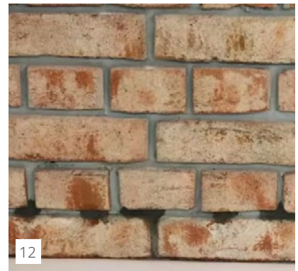
12 The drill holes are sealed with KÖSTER KB-Fix 5.
